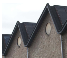
RONDE OPENING IN NOKKEN SHEDS
